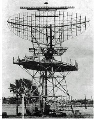
OVERVIEW: The AN/FPS-66 is fixed, long-range, L-Band General Air Surveillance Radar
