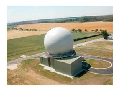
Sensors / EW: - HR-3000 - (HADR) Radar, Radar, Air Search, 3D Long-Range, Max range: 500 km
