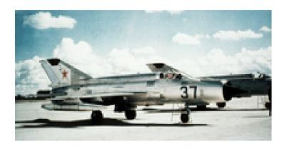
Sensors / EW: - Jay Bird [RP-22M Sapfir-21] - Radar, Radar, FCR, Air-to-Air, Short-Range, Max range: 29.6 km - SPO-10 Sirena-3M - ESM, RWR, Radar Warning Receiver, Max range: 222.2 km
